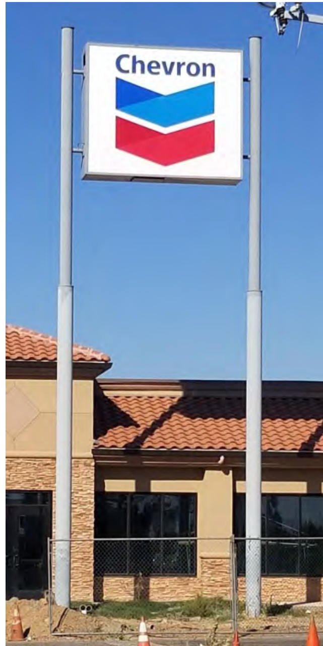
EXISTING 40'-0" PYLON TO BE REMOVED
